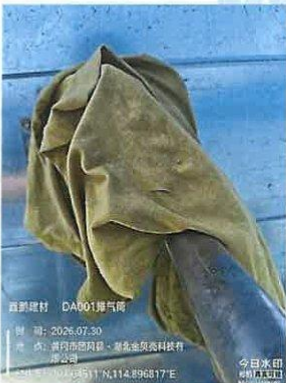
◎4称重预混粉尘废气排气筒DA001
