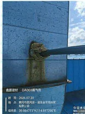
◎6抛光废气排气筒DA003
